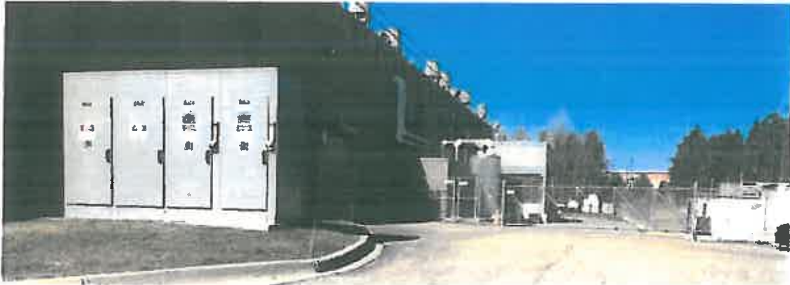
EQUIPMENT IMMEDIATELY ADJACENT TO WEST PROPERTY LINE OF BECK ROAD RESIDENCE HOTEL SITE
